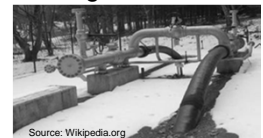
Pig Launcher
