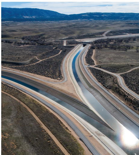
The California Aqueduct bifurcates as it travels into Southern California.
